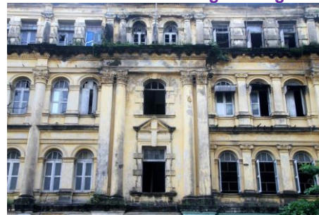
Old British Office Building in Yangon
